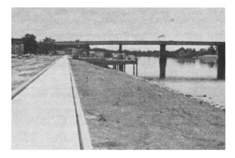
a. Floodwall in the collapsed position
