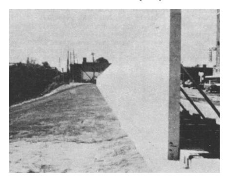
b. Floodwall in the raised position
