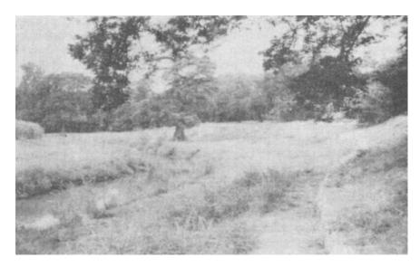
Figure 4-8. Vegetative lining, San Antonio River flood channel (USAED, Fort Worth). This completed reach contains a subchannel that conveys normal flows. The high-flow berms and banks are vegetated. Note the River Walk (Paseo del Rio) inside the flood channel
